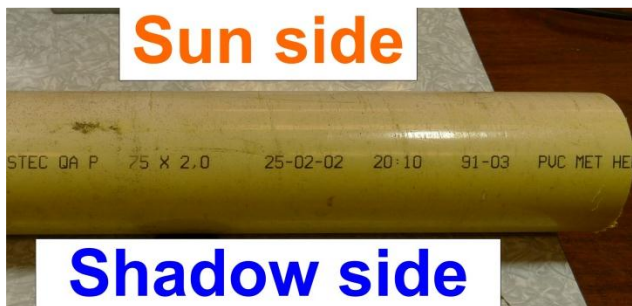
Figure 8: PVC pipe where the discolouration of the sun side is visible.
