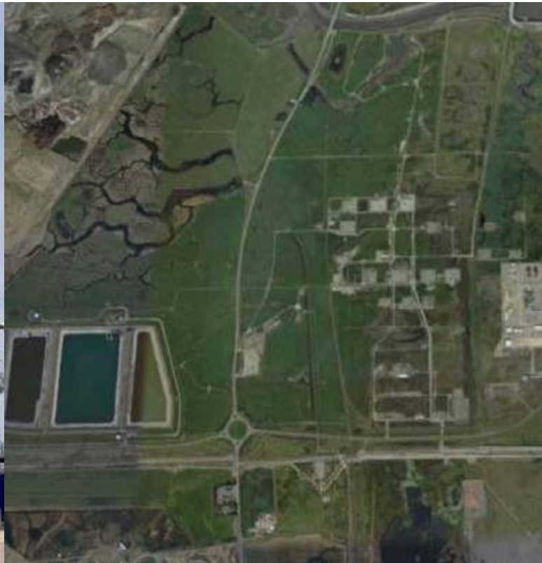
Image 2.4. Existing BOC 36.4 MMSCFD (c. 150 MW) SMR at Teesside
