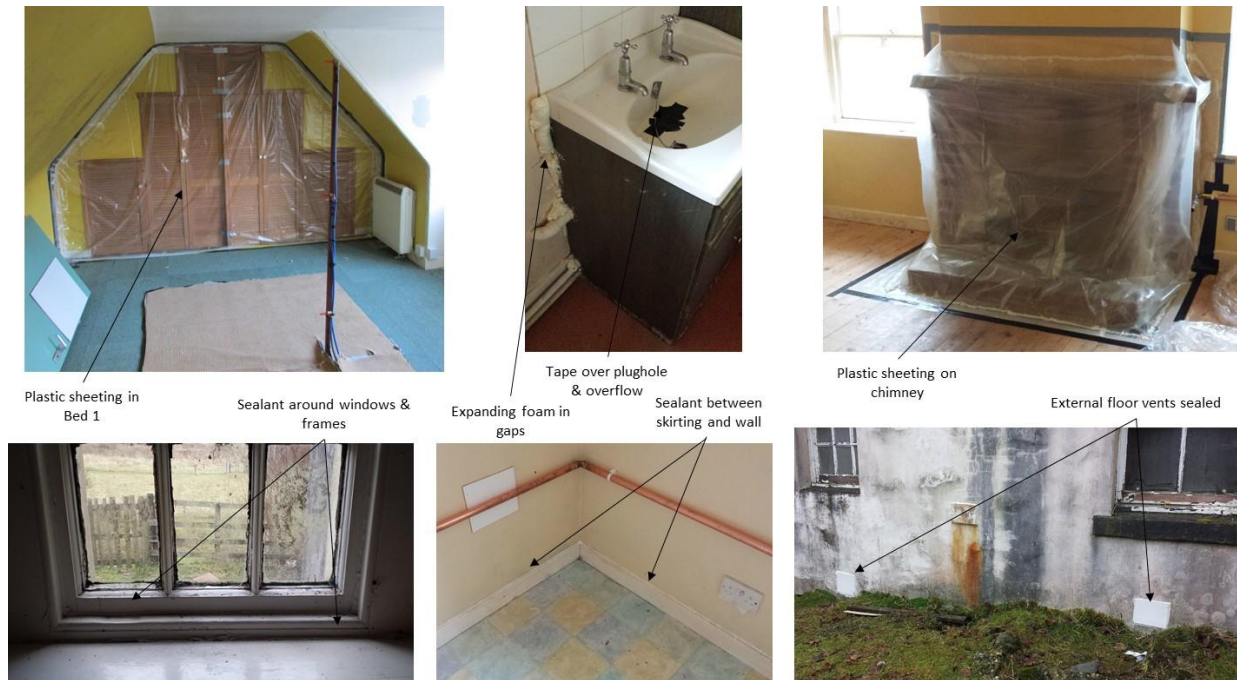
Figure 12: Examples of sealing measures after phase 1 and before phase 2
