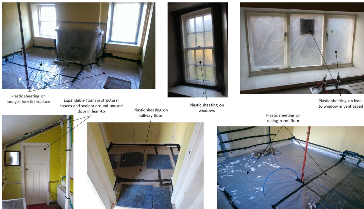
Figure 13: Examples of sealing measures after phase 2 and before phase 3
