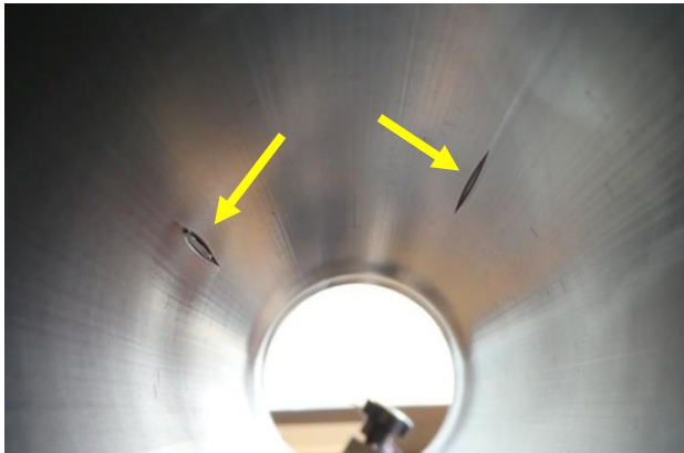
Figure 6. Pipe failure after testing in the horizontal container. Two cracks are visible at the top of the pipe (yellow arrows), although only one has failed.
